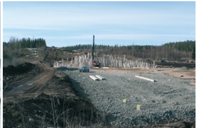
Figure 22. Piling through the mass stabilised soil
