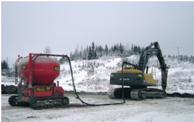
Figure 22. Stabilisation were carried out also in winter
