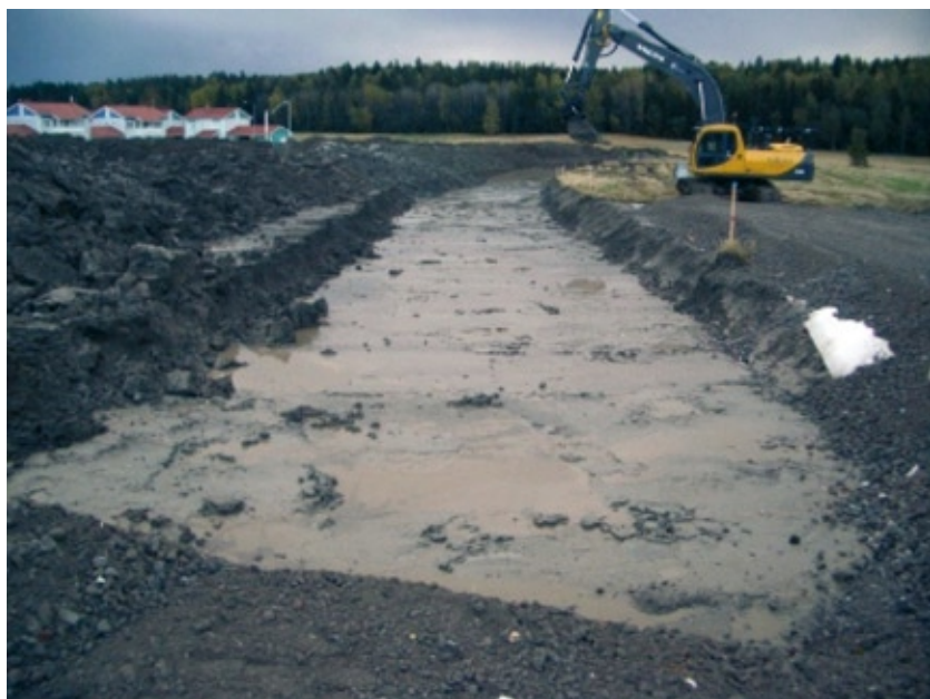
Picture: Mass stabilisation in a residential area.
