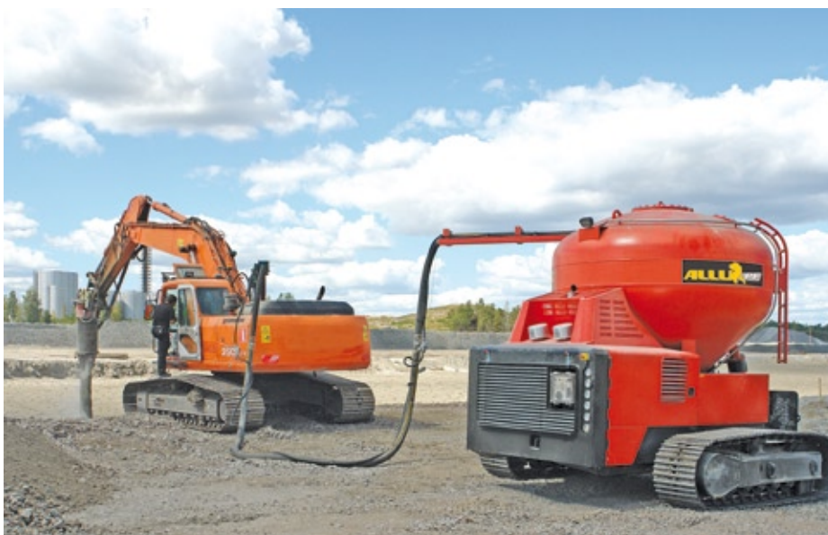
Picture: ALLU Stabilisation system at work
