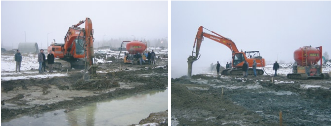
Figure 27 and 28. Stabilisation of soil for residential area in Kirkkonummi, Finland.
